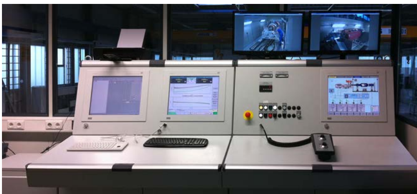
Control room of a high-speed balancing and over-speed testing installation
