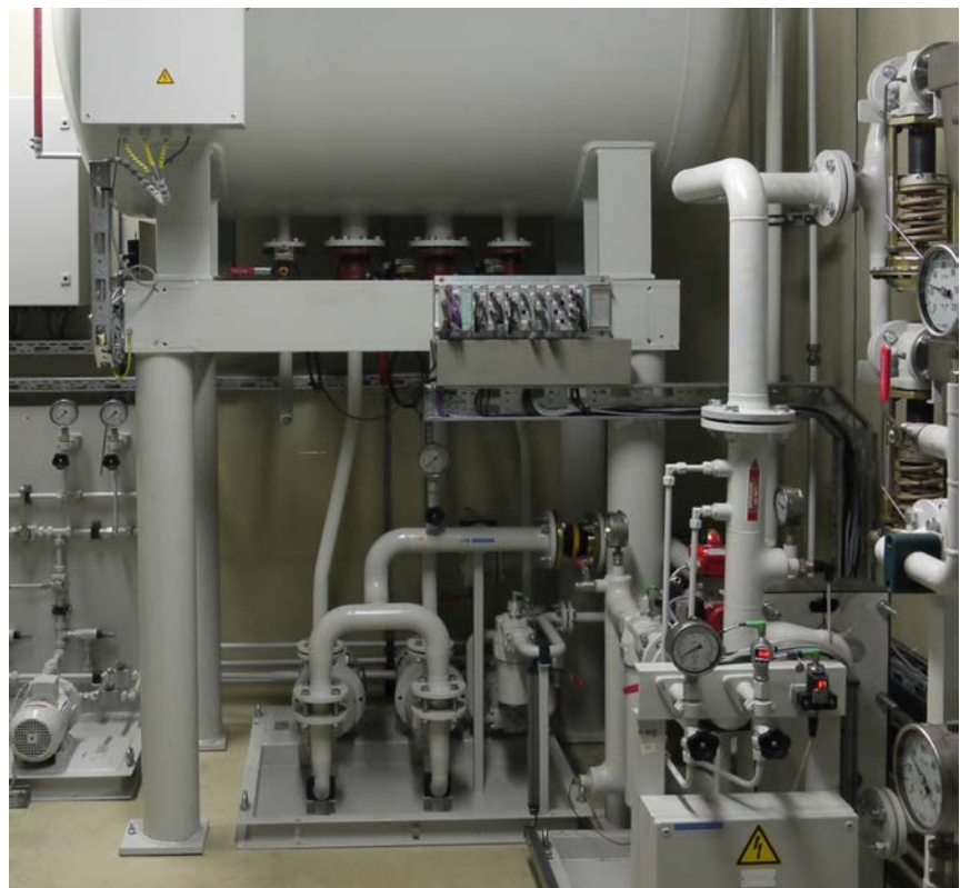
Vacuum oil station, installed underneath vacuum oil tank, and vacuum oil distribution with filtering, flow monitors and pressure control
